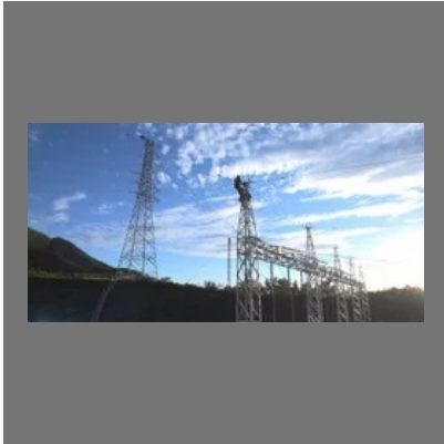
Opgw Installation Services
